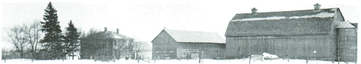
Francis Homestead at Northcote in Admaston Township, Renfrew County Photo Taken December 25, 1934
